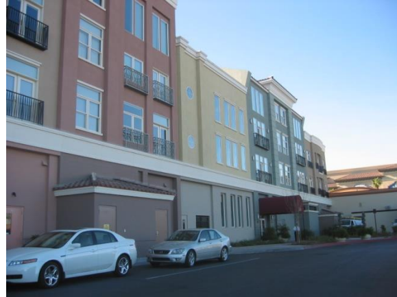
Figure 6-16: This figure shows two methods of using architectural features to create wall surface relief on wall elevations that are not the primary elevation.
